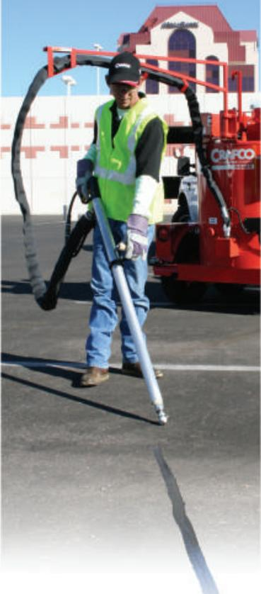
Pavement is a costly investment. Just as you would seal leaks in the roof of your building you should seal cracks in your pavement. Water infiltration through cracks causes deterioration of the pavement and substructure. Untreated cracks propagate and multiply, developing potholes. The result is expensive repairs and reconstruction.
